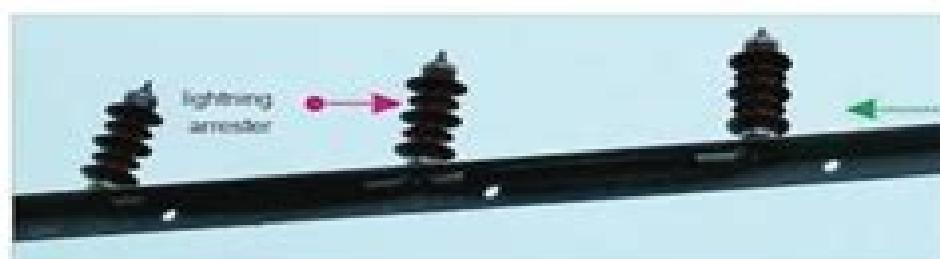
Lightning arresters are sometimes called over-voltage protectors, which are mainly used to protect electrical equipment from high transient over-voltage hazards, that is, from damage caused by lightning over-voltage and operating over-voltage.
